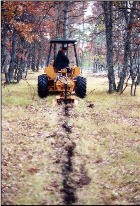
Figure 19. Vibratory plow trenching.
